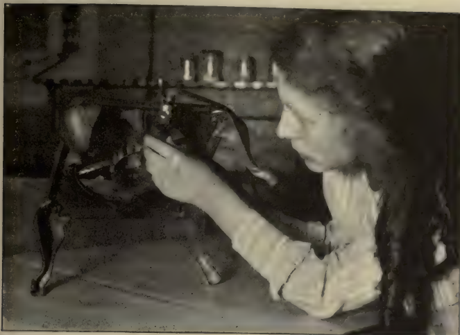
FIG. 169. Regulating the air opening in a gas stove.
